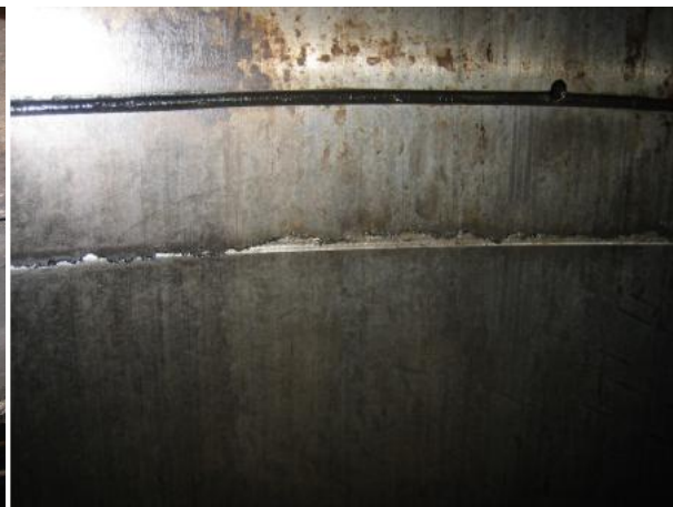
Cracked cylinder liner
